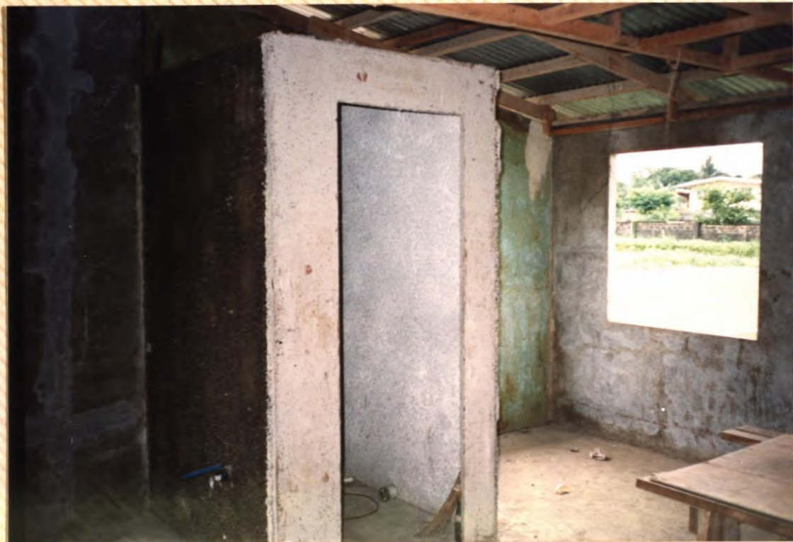
No. 45. Unfinished bathroom enclosure of MKL-33 House.
