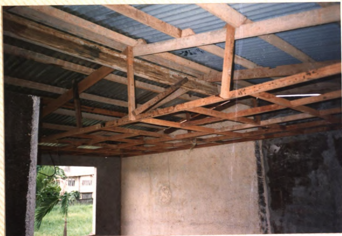
No. 46. Unfinished ceiling framing of MKL-33 House.
