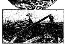
The photos above, taken after the preat fire had passed through frequois Falls, give some idea of the terrific heat all around the Abitibi Pulp & Paper Co. plant. Note the bent and twisted steel rails and frame-work.
