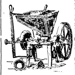
This is our Grinder to run with a tread power or other light motive power. Notice the two balance wheels to hold the speed steady. It will crush and grind shucked corn as well as all sorts of small grain. Notice the conical grinding plates. We make two sizes larger also. SEND FOR CATALOGUE.
