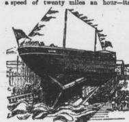
LAUNCH OF THE YORKTOWN. shape being calculated for speed-it is plain that the destroyer can "shoot and run," like the militia captain of the old story. The engines are toward the stern. triple expansion machines developing 3,300 horse power, to both run the ves
