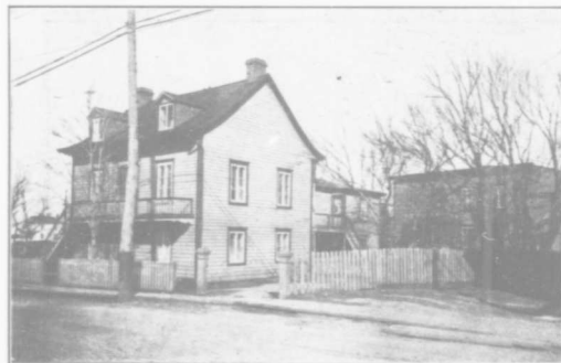
GEORGES ROY 60 Fraser General Contractor Entrepreneur Général
