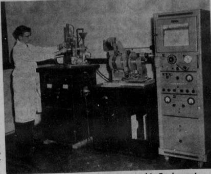
X-ray Defraction and Spectrographic Equipment
