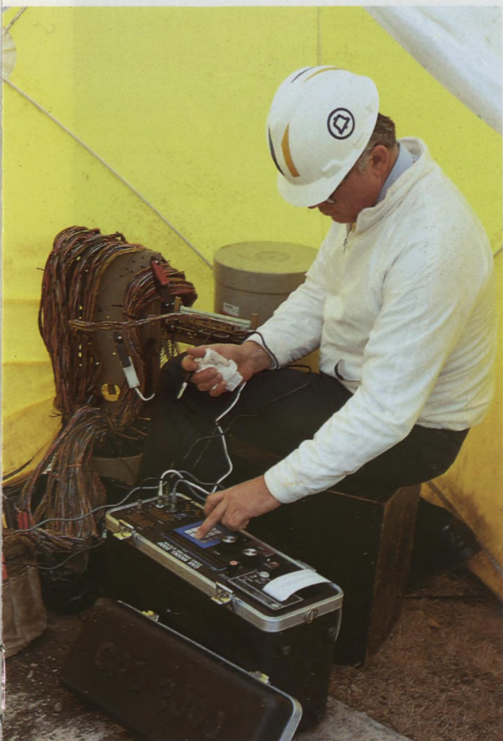
COMMUNICATIONS TECHNOLOGY (CANADA) LTD.
