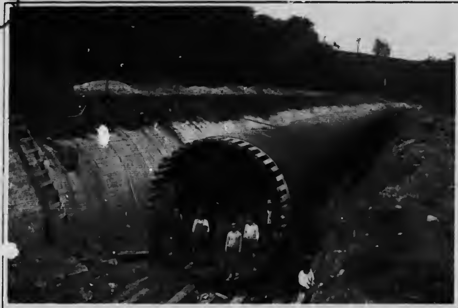
Wood Stave Pipe Line during Construction.
