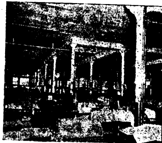
After Luxfer Prisms Installed.
