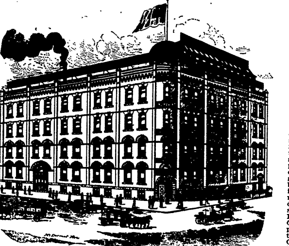
The New Stovel Block, Winnipeg.
