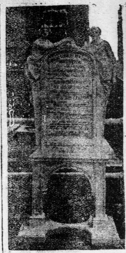
Bulletin Board Outside the New Suffrage Headquarters.
