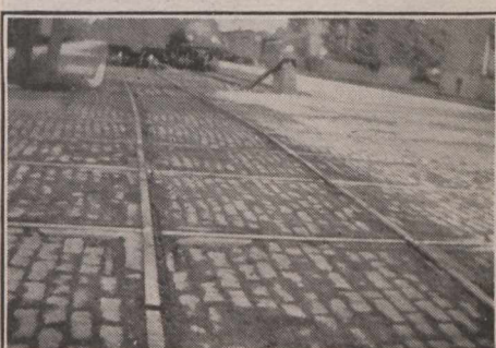
Trussed Rail Joint, London Street Railway.
