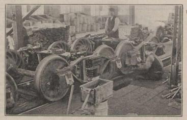
Fig. 4.—Final Step in Car Truck Assembling.
