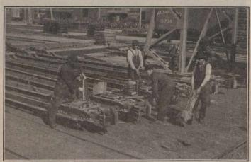
Fig. 5 .- Fitting Draft Gear into Centre Sill.
