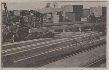
Fig. 6.—Rivetting Centre Sill to Body Bolster.
