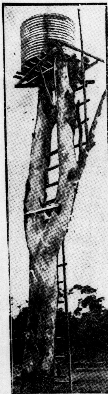
W. Showels of Brookvale, Australia, has put his water tank on the top of this old tree.
