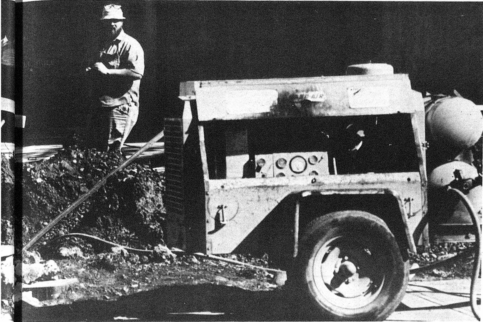
thundering jackhammers was commonly heard during the early days of September as construction crews wrapped up a summer's work. Above Bob McGregor of the plant checks progress on the sprinkler system on the east side of SUB.
