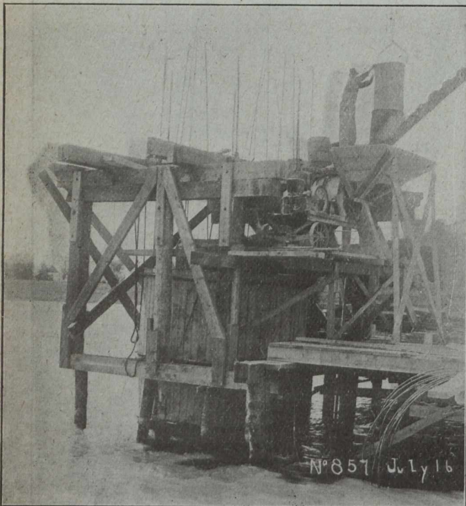
Concreting a 6 ft. Caisson Lift
