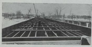
View of Bridge Under Construction, Showing Floor Beams and Stringers.
