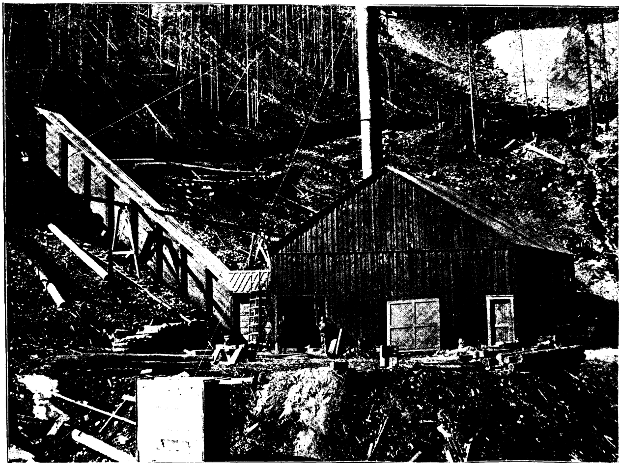
WAR EAGLE COMPRESSOR PLANT, ROSSLAND, B.C.
