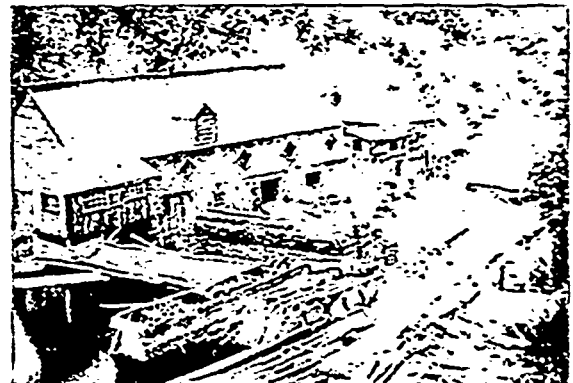
ROTARY AND GANG MILL AT WHITE ROCK.
