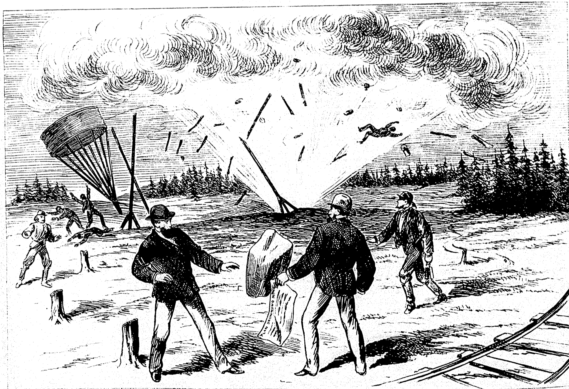
THE "BLOW" FROM THE PUMPING SHAFT.—DEATH OF BURNS AND NARROW ESCAPE OF MEMBERS HUDSON AND COXON.
