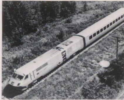
1,096 miles in an 11-hour shift with an average speed of 93.6 miles per hour, with three station stops for crew changes. It also showed a remarkably low level of fuel consumption, averaging 0.8 US gallons per mile over the 20,700 mile test run.
