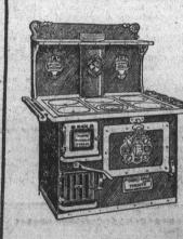
The Oxford Chancellor Range, though built with durability and strength as the primary objects, is very handsome in appearance. The ornamentation is very plain and solid so that it is easily kept clean. The top edges and door frames are nickle-plated.
