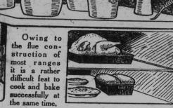
But the arrangement of the Pandora flues differs considerably from others. They are so constructed that the draft for baking is also the best for cooking, the heat circulating around the oven twice and under every pot hole before passing up the chimney.
