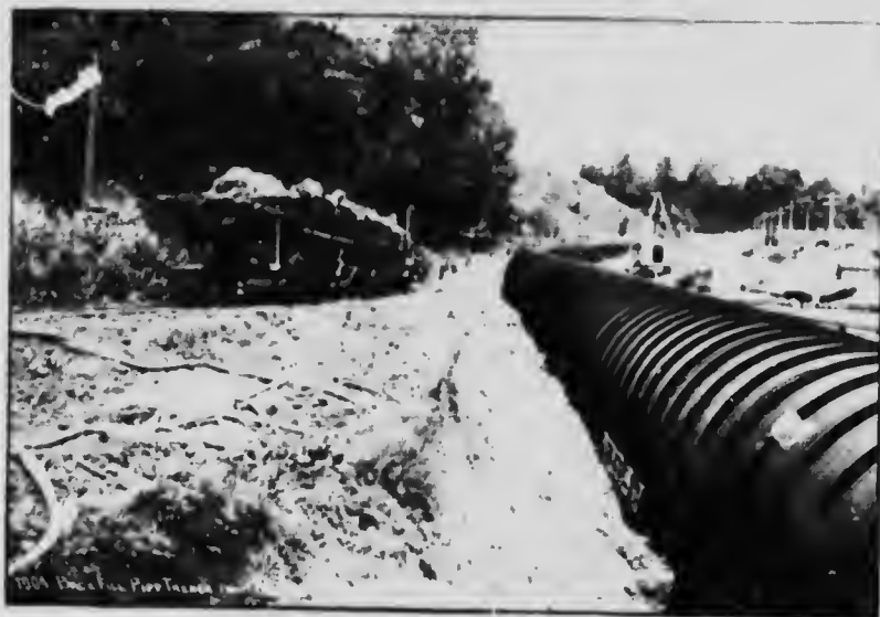
ONTARIO POWER COMPANY, MAIN CONDUIT EIGHTEEN FEET DIAMETER
