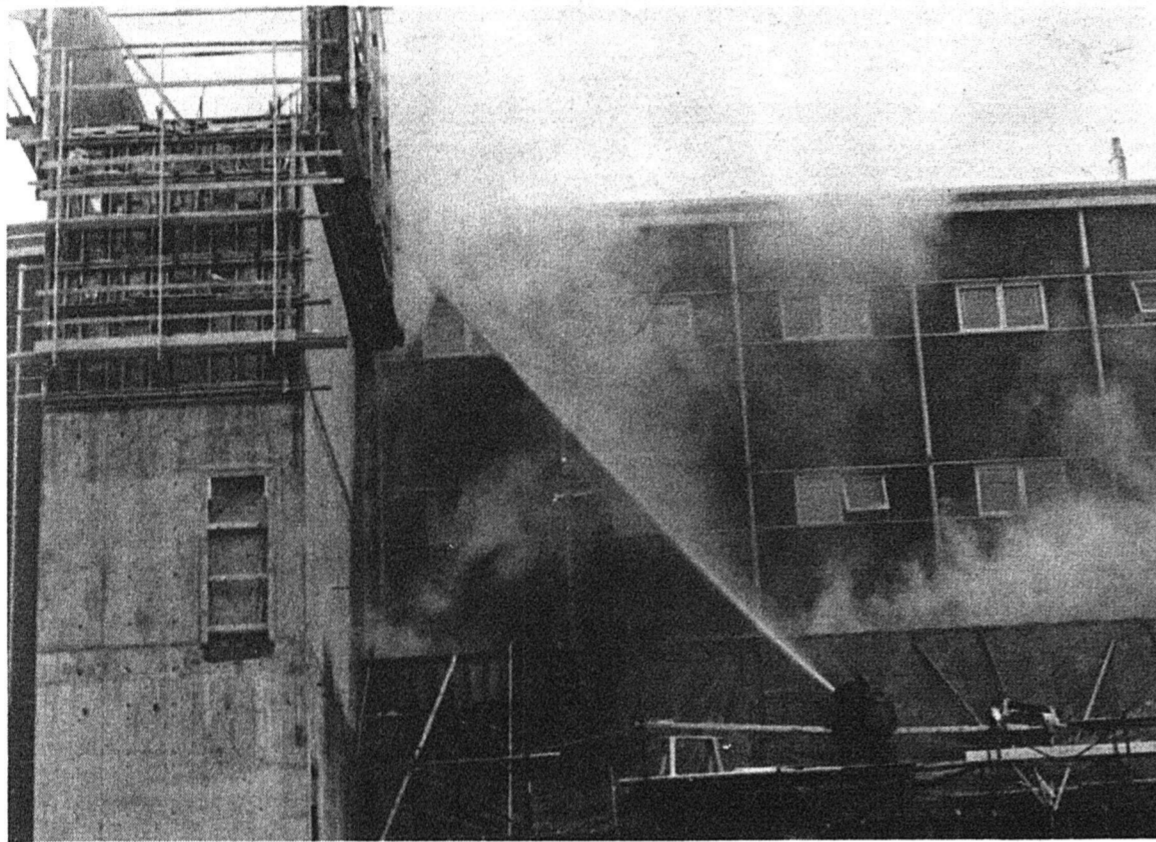
When gas escaping from a number of propane tanks caught fire and set aflame rubbish around them, this was the result. The construction next to the chem building was the scene of the fire. No serious damage seems to have been done. However, the fire was very near an undergrad chem lab; so there was potential for considerable damage.
